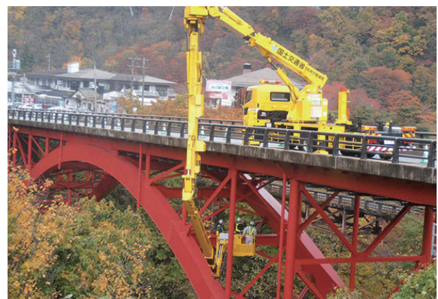
Fig. 2 Inspection of an arch deck bridge 4)
