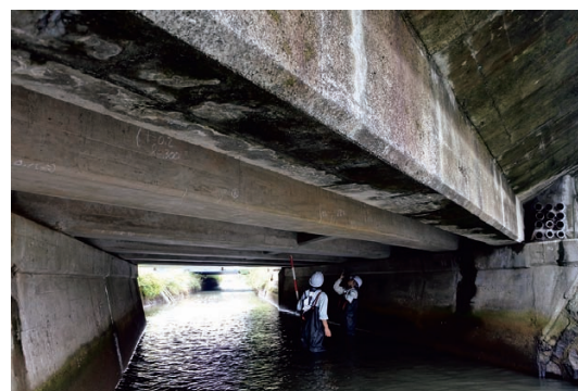
(b) From under the girder
