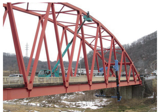
Fig. 1 Inspection of a trussed Langer bottom-road bridge 4)
