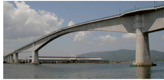
Fig. 3 Eshima Ohashi Bridge
