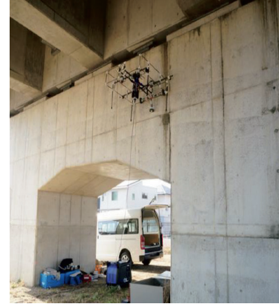
Fig. 8 Inspection of the side of a pier.
