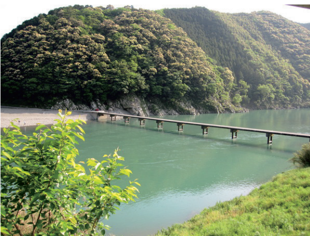
Fig. 1 Iwama Ohashi bridge before collapse
