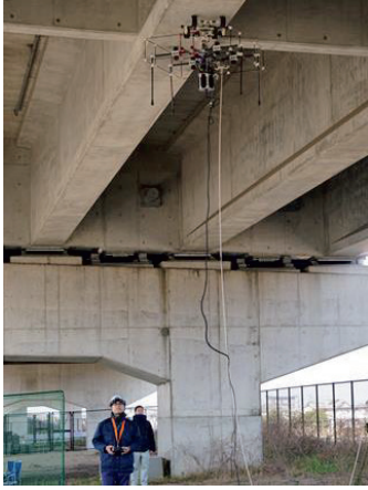
Fig. 6 Inspection of the area under girder.
