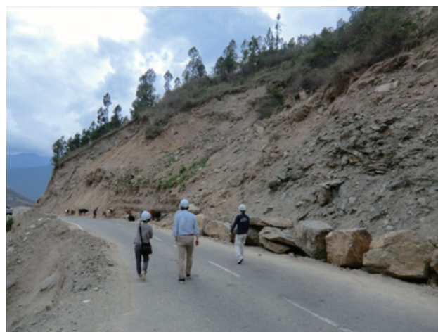
Fig. 1 Slope collapse on National Highway 1 in Bhutan
