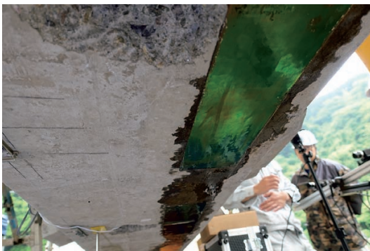
(b) Installation of the measurement device
