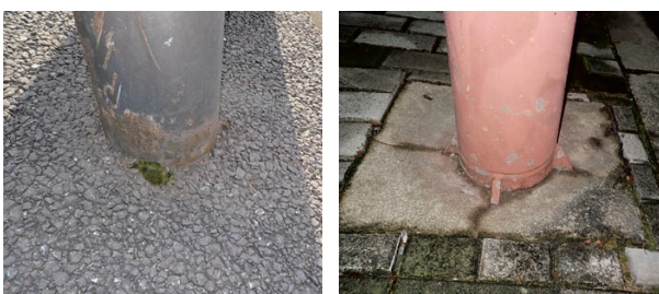
Fig. 1 Embedded portions of the bases of light poles and signposts
