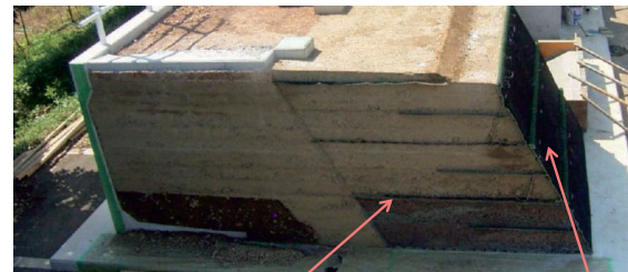
A slope surface is formed with metal mesh.
