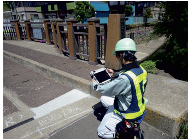
Fig. 5 Bridge inspection using a tablet terminal
