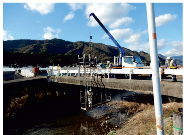
Fig. 2 Similar needs of different local governments: Demonstration of simple inspection scaffolding (left: Kinki Forum, right: Ehime University)
