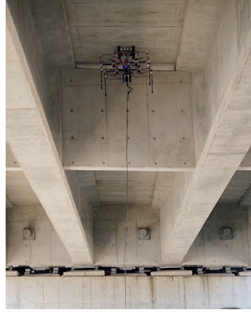
Fig. 7 Inspection of the deck.
