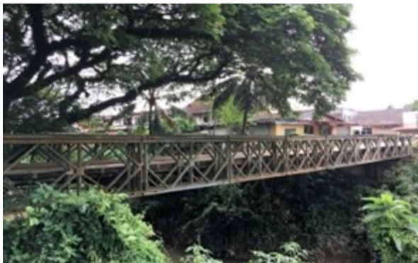
Bridge B (ラオス)
