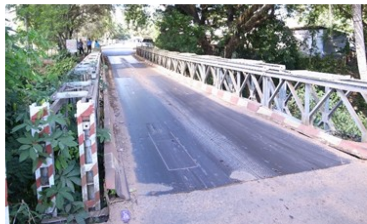
Bridge B: Steel plates
