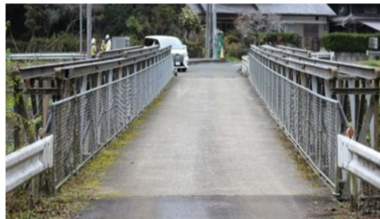
Bridge D: Concrete
