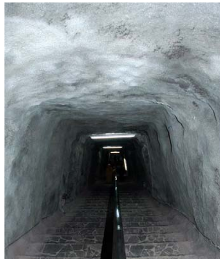
(b) View of inclined shaft
