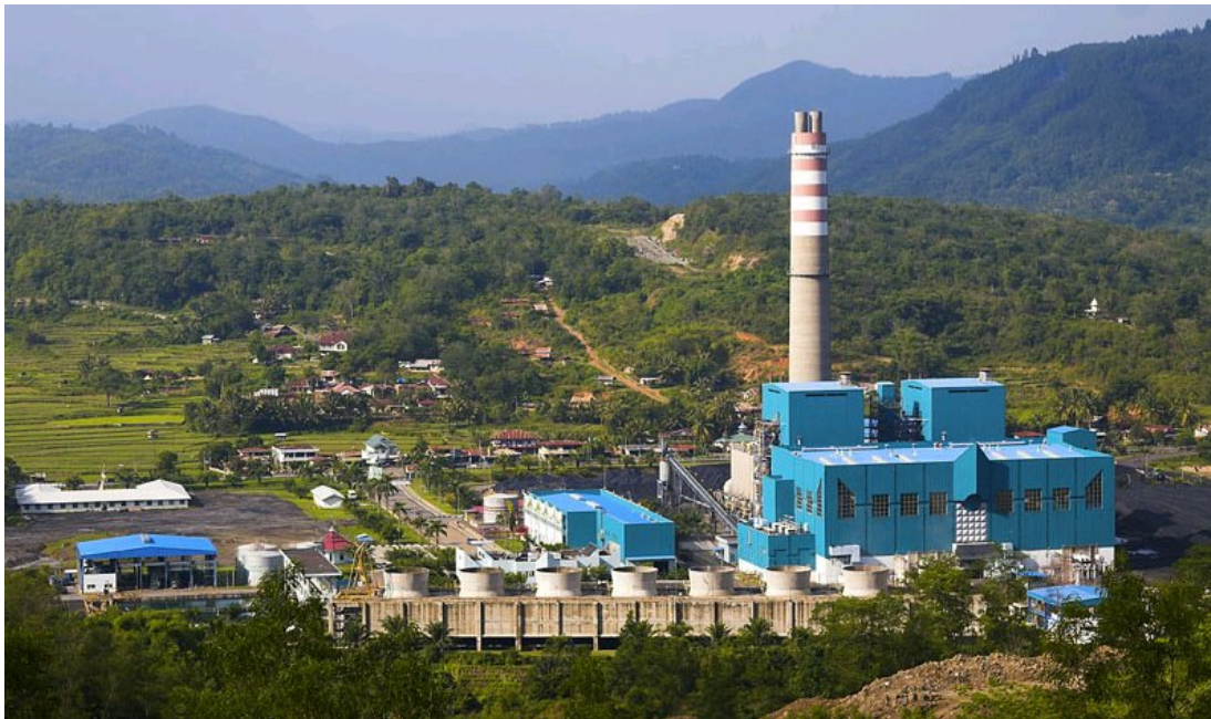
Figure 10.4. A view of Kandi Thermo-electric Power Plant
