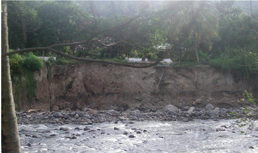
(a) Embankment failure at Sumpur Village (the nearest site to the epicenter)
