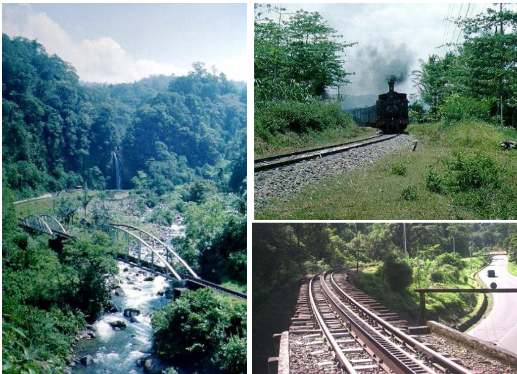
Figure 6.1. Views of railway lines in the epicentral area
