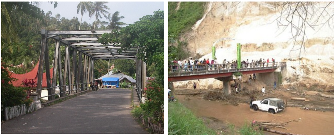
(a) Truss bridge in Sumpur village
