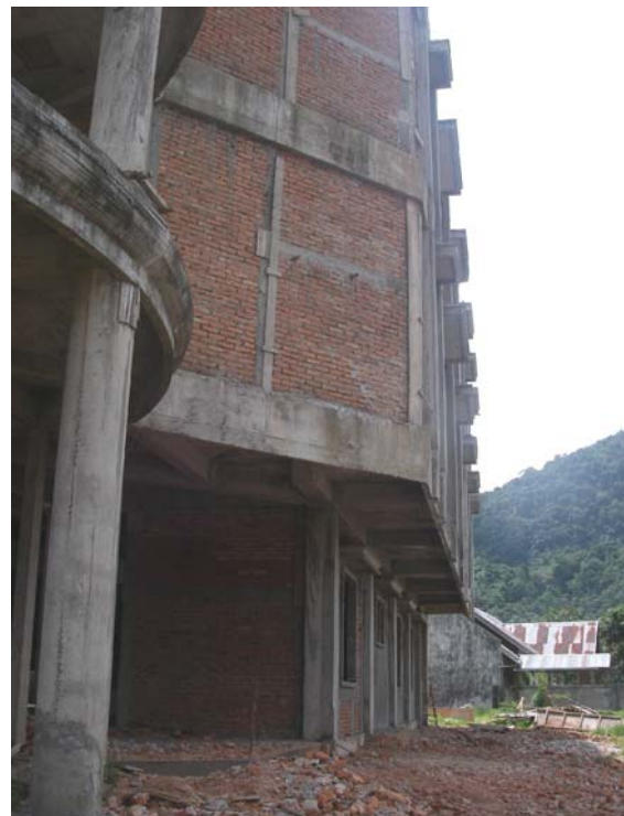
(e) Slightly damaged RC buildings in Padang Panjang
