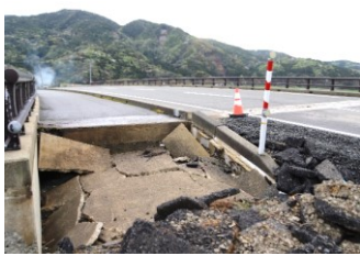
(c) Step at approaches to bridge
