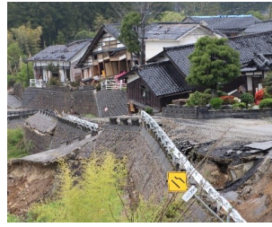
(b) Ground deformation occurred in vicinity of bridge
