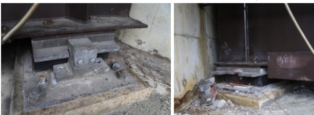
(c) Damage to attachment of rubber bearings
