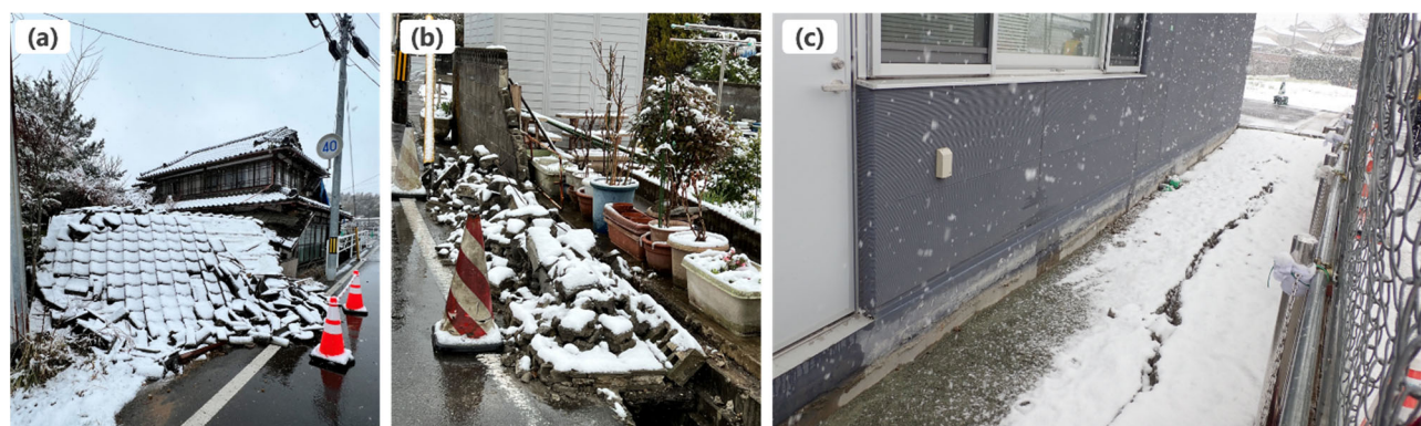
Fig.16 (a) Collapsed house (old residential area), (b) collapsed concrete-block wall (old residential area), (c) ground crack in the vicinity of the Center (newly landfilled area)
