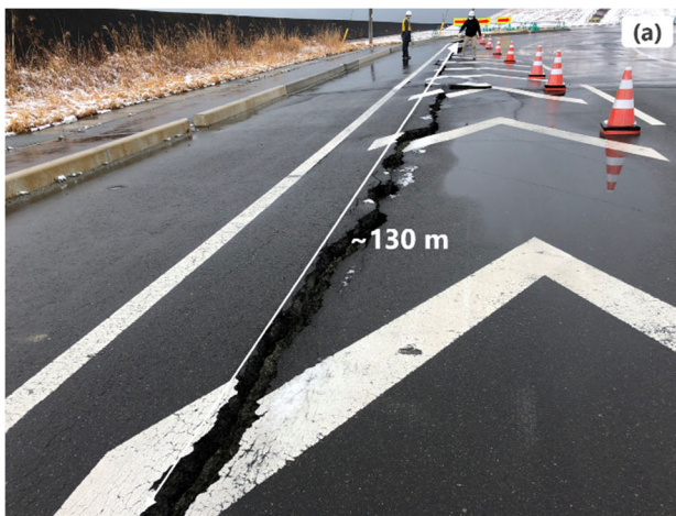
Fig.9 (a) a 130m-long crack on the carriageway in Quay No. 5, (b) Coal unloading machine with ruptured transverse beam
