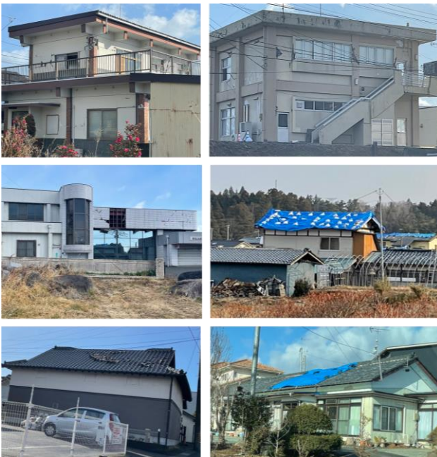
Photo 13 Representative damage to house in Shinchi Town.
