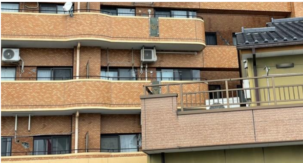
Photo 12 A residential building with SRC structure in Fukushima City. (south elevation, east-west orientation)
