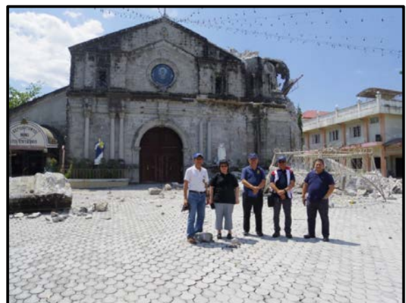
Fig. 12. Bell Tower damage to Santa Catalina Church
