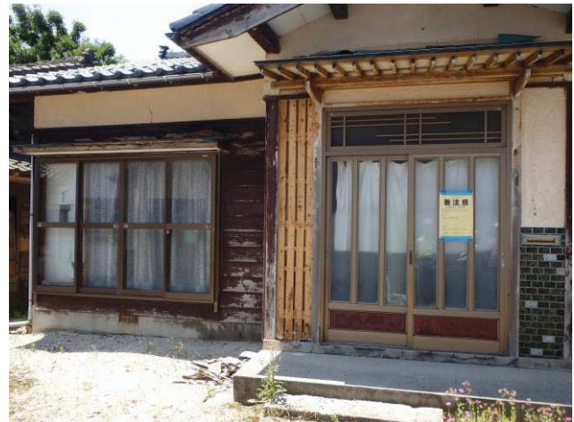
Photo 8 Damage of exterior building material of old wooden house in Fuya area (N38.516733, E139.534405).
