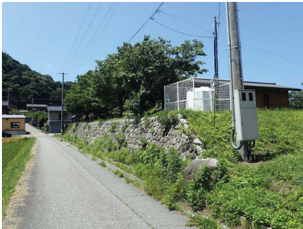
Photo 1 The seismic station of NIG006 that observed seismic intensity 5- (N38.45075, E139.496175).
