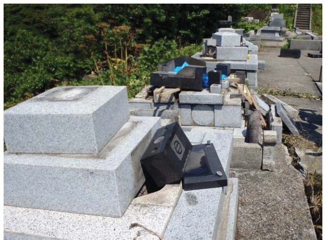
Photo 11 Damage of tombstone at Koiwagawa (N38.589553, E139.565355).
