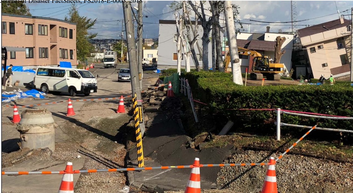
Fig. 9 Swath of ground subsidence in the boxed area in Fig. 7 (Photo taken on Oct. 8, 2018 at N42.9890°, E141.4555° by Daiki Kodama)
