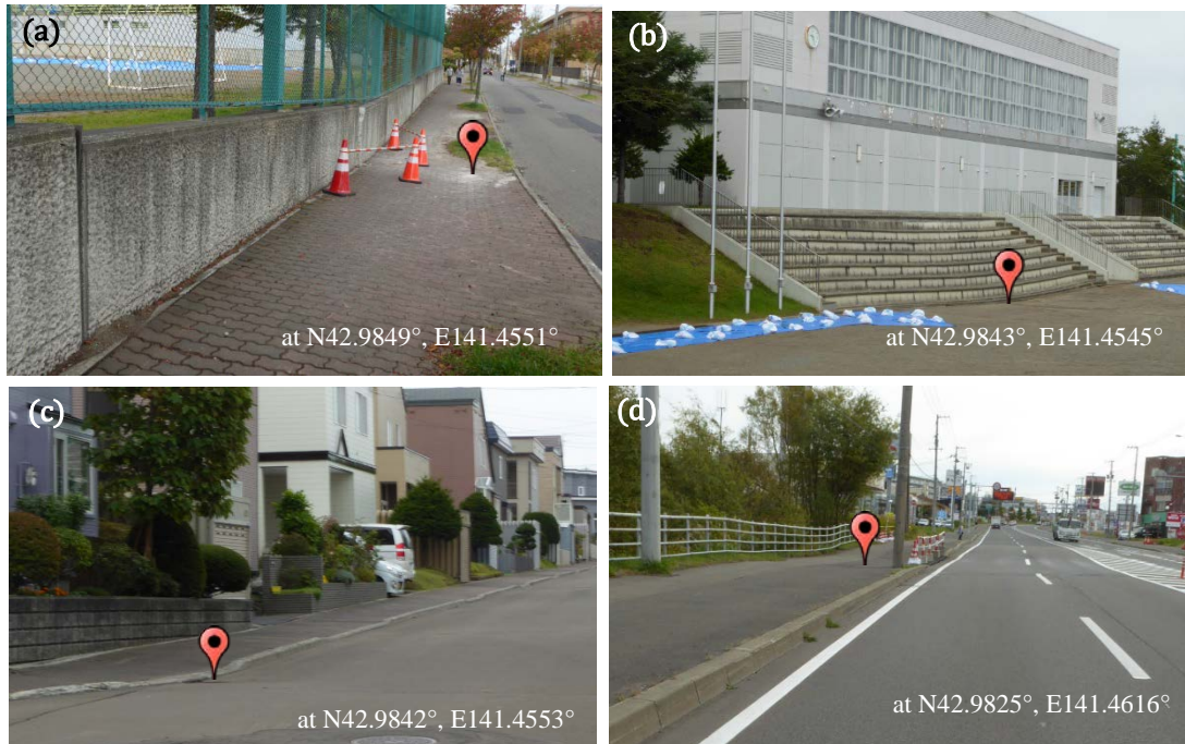
Fig. 10 Sunken roads in Sapporo's Kiyota Ward (Photos taken on Oct. 10, 2018 by Kazuo Konagai)
