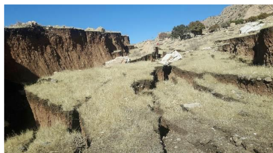
Photo 2 Ground subsidence close to Mela Kabood village
