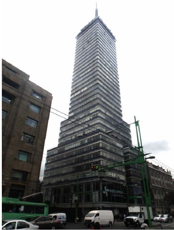
Fig.11 Latin-American Tower, D0, Zone III
