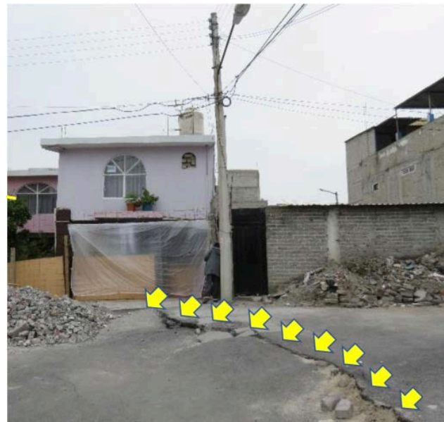
Fig.25 Site 2. House with a sinkhole
